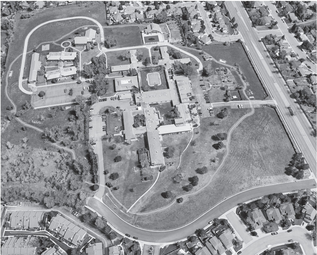
Fig. 19.4. Aerial view of the 31-acre Oxford Vista site in Aurora, Colorado.
